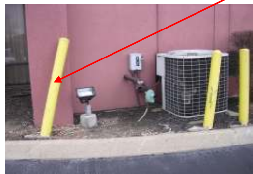
All 8 bollards are loose and no longer vertical.
