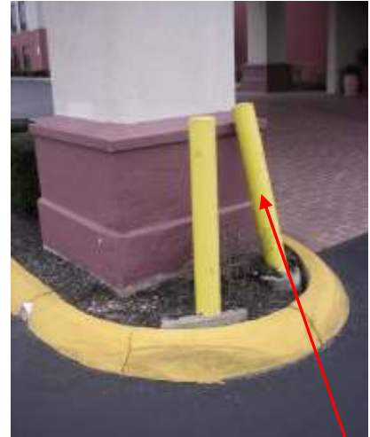
All 8 bollards are loose and no longer vertical.
