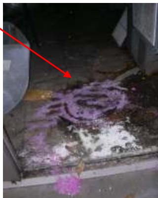
Caused floor of room for HVAC units 1E, 1F, 1G, 1I, and 1H to be soaked, and water drained to conference room.
