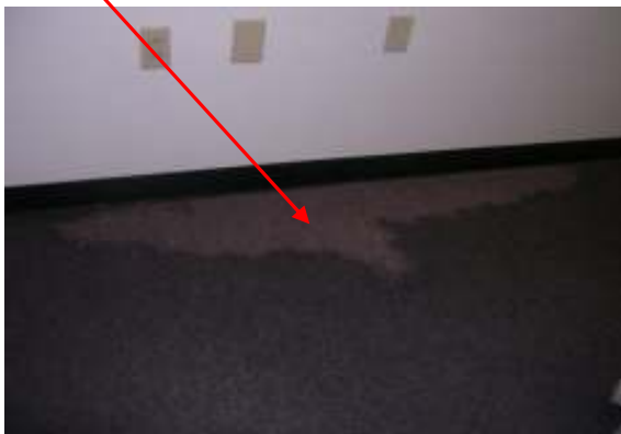
Caused floor of room for HVAC units 1E, 1F, 1G, 1I, and 1H to be soaked, and water drained to conference room.
