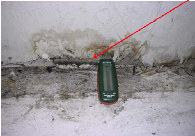
The OSB wood wall at the rear of the second warehouse was holding as much moisture to peg the moisture meter (above 44%).
