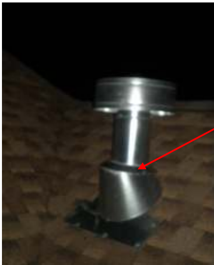
Pieces separating. Water will come into the attic.
