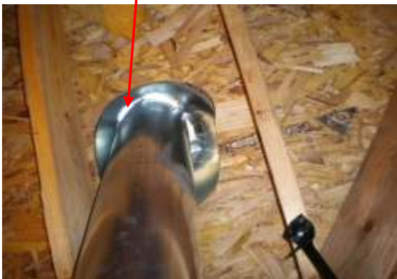
Pieces separating. Water will come into the attic.
